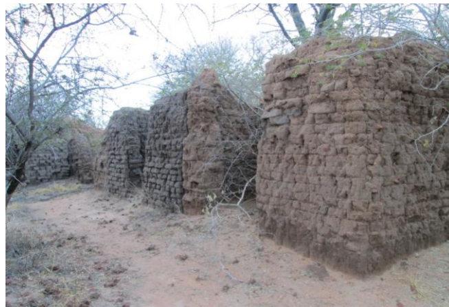
Figure 35: Mission Station ruins, indicating the red sundried and grey wood fired bricks (Photograph by author 2018).
