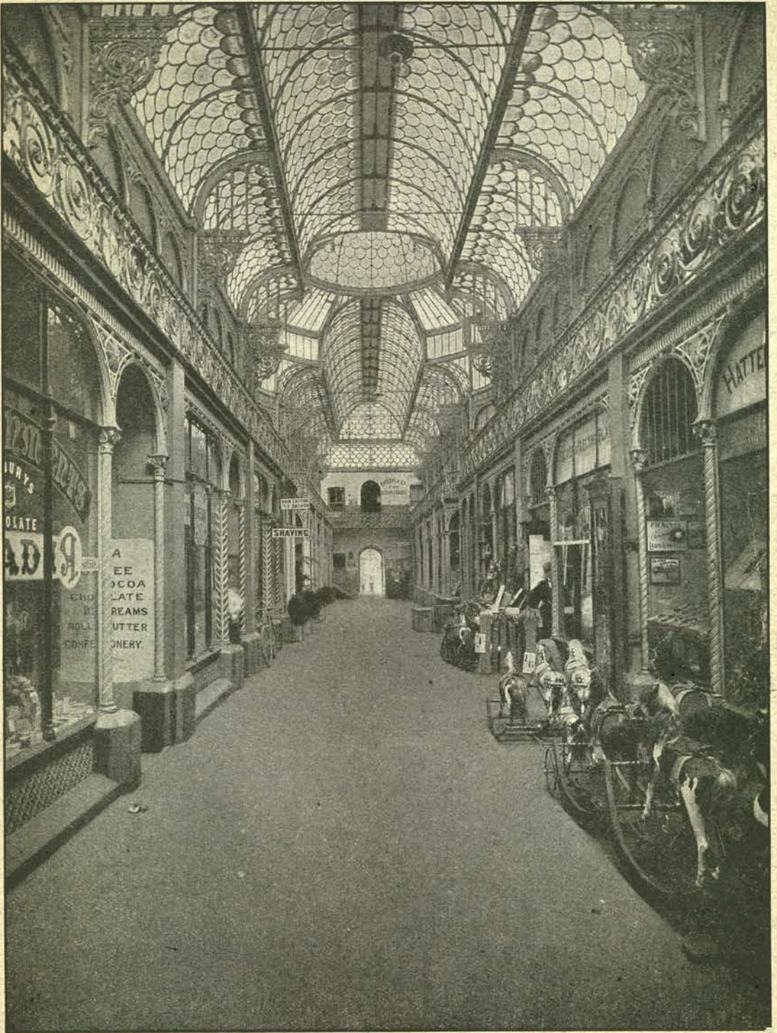
ARCADE ERECTED BY US AT JOHANNESBURG
