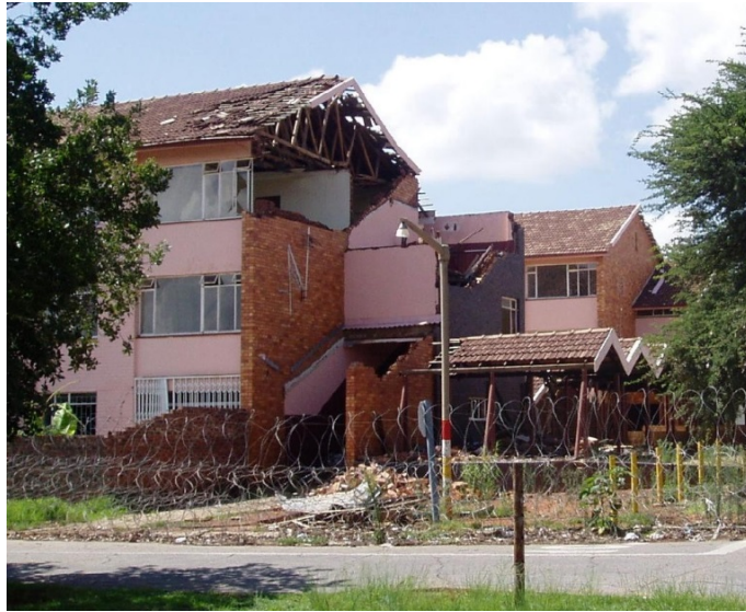
Figure 5.7: Damage following the Stilfontein earthquake of 2005 (Durrheim et al. , 2006)
