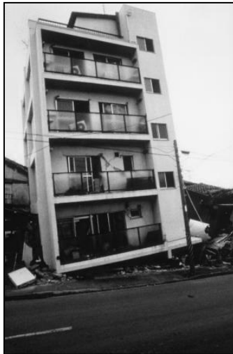
Figure 2.4: Building class 8, reinforced concrete shear wall, without moment resisting frame, medium rise (EMS, 1998)
