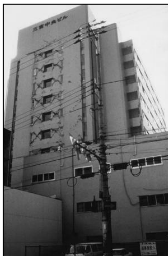
Figure 2.5: Building class 9, reinforced concrete shear wall, without moment resisting frame, high rise (EMS, 1998)
