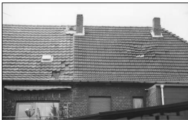
Figure 2.2: Building class 3, unreinforced masonry, with load bearing wall, low rise (EMS, 1998)
