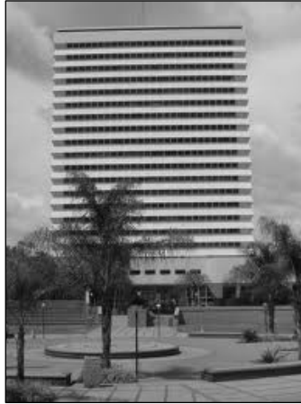
Figure 2.3: Building class 7, reinforced concrete shear wall, with moment resisting frame, high rise (panoramio.com, 2008)
