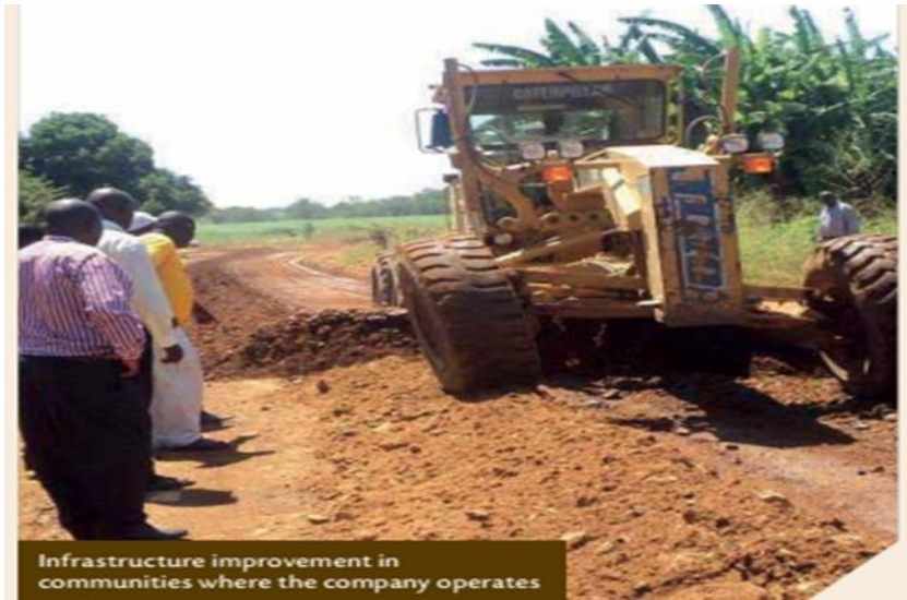
Figure 7-8: Road construction to improve infrastructure in communities
