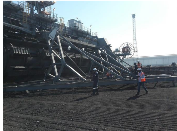
Figure 75 Rake failure side view
