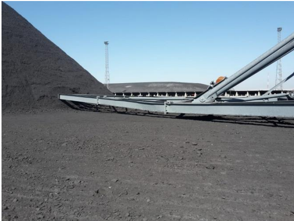
Figure 74 30 ton rake failure
