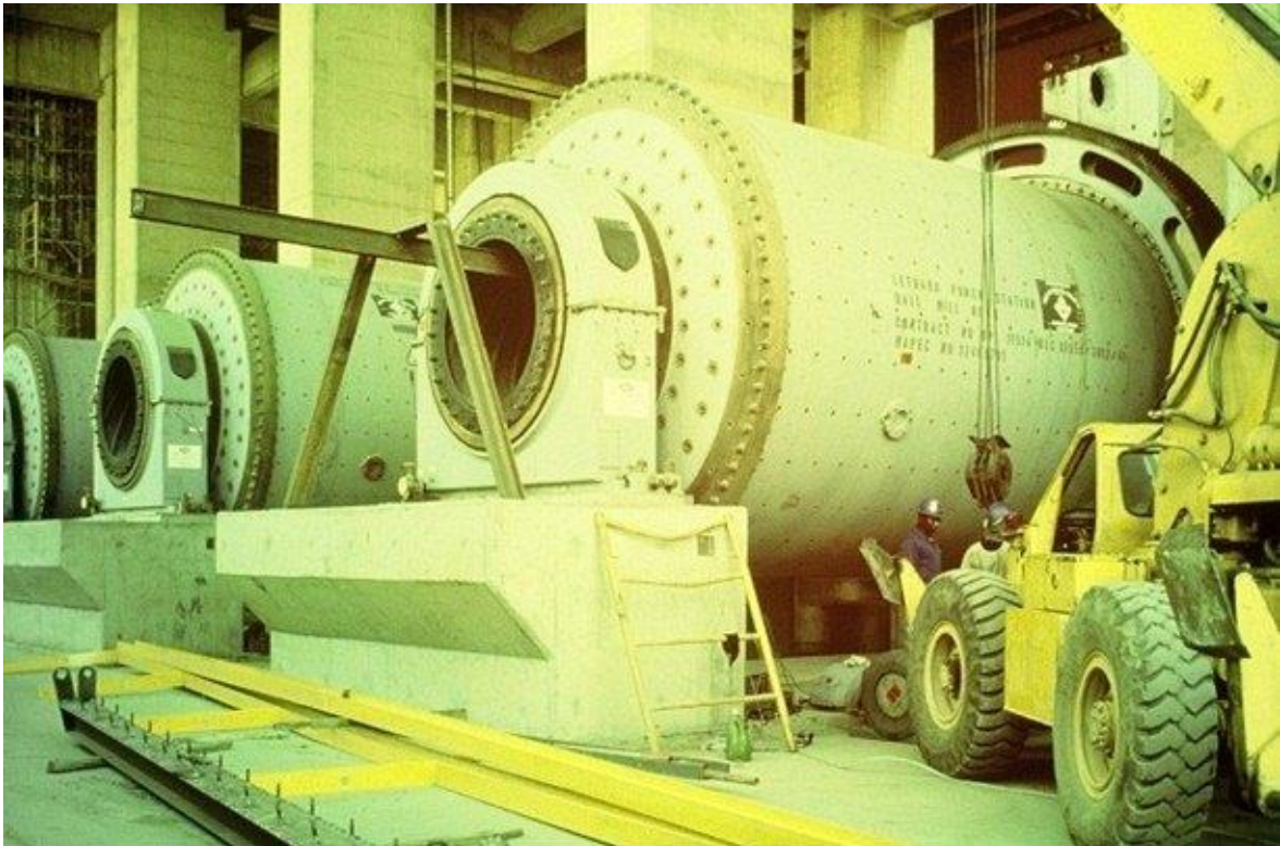
Figure 45 Lethabo Power Station ball mills being installed
