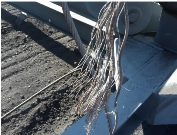
Figure 76 Wire rope failure that lead to rake collapse
