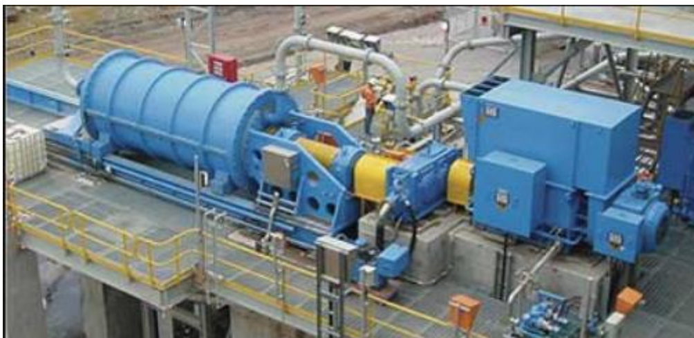
Figure 4: Picture of an IsaMill installation, www.isamill.com 2018
