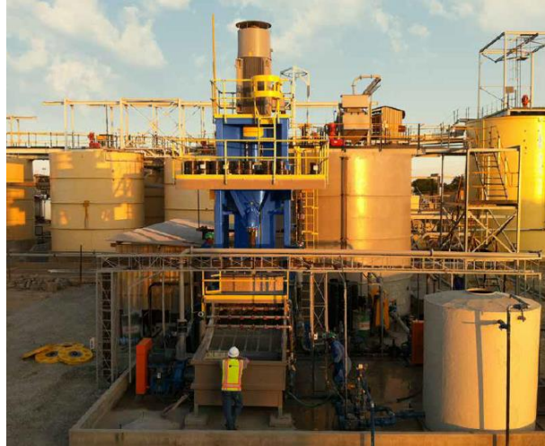
Figure 13: Picture of an industrial VXP mill installation, FLSmidth 2018
