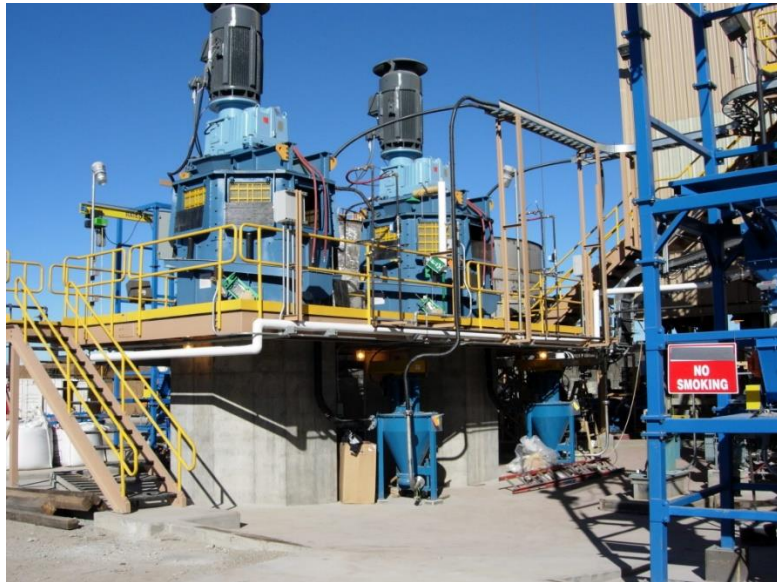
Figure 7: Picture of an SMD installation with two mills, www.metso.com 2018
