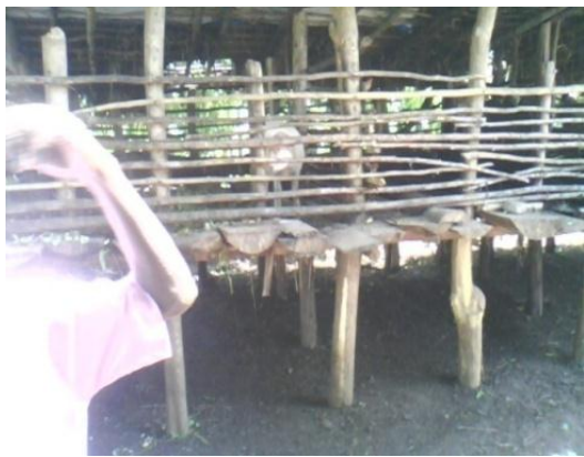
Figure 2-5: Pig pen built off the ground.
