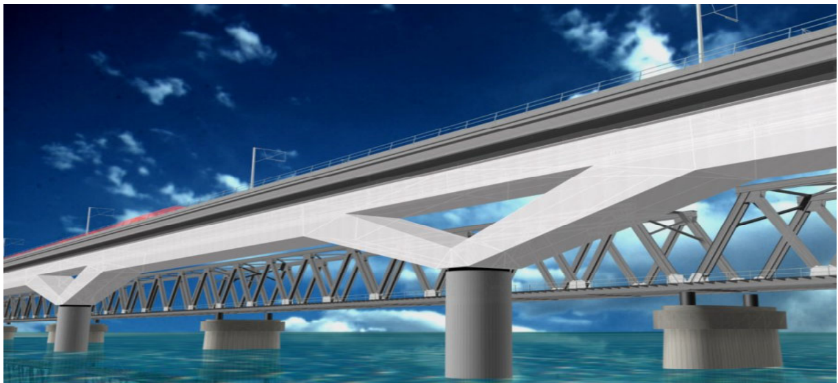
Figure 5: Hollandche Diep Bridge
