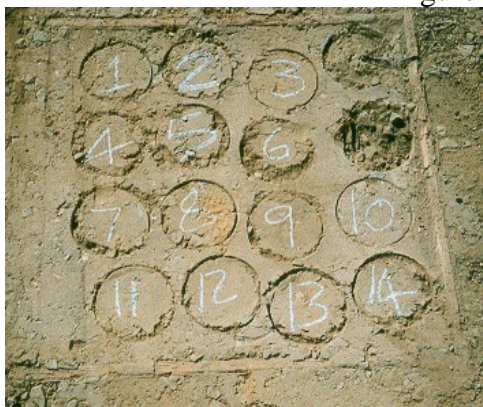
(a) G2 slab after coring
