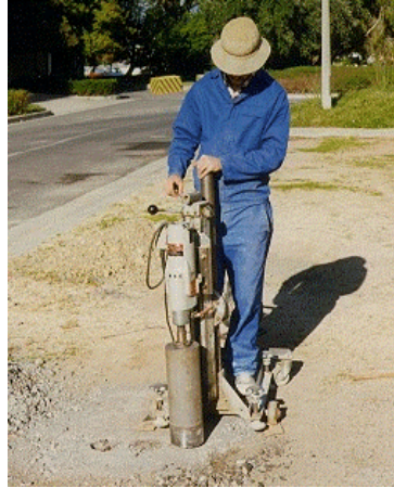
Figure 2: Coring in progress
