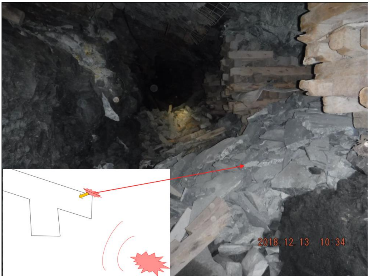
Figure 32. Observed strain burst from south siding corner with hanging wall.
