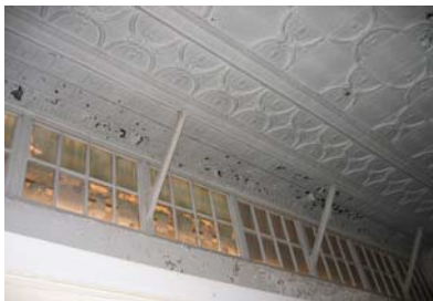
Fig. 2.10: Pressed steel ceiling found in the east wing (Photographs by Niebhur (2008))
