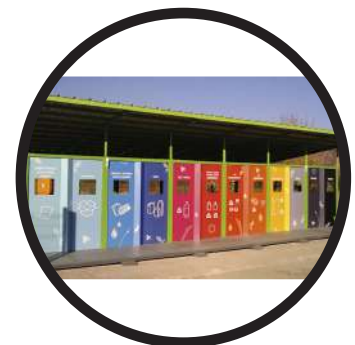
Fig 4.54: Waste collecting infrastructure
