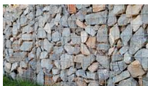
Fig 8.13: Natural stone in gabion basket Locally found material connecting man with the natural elements and allow for multi sensory experience ,ease of maintainance and wayfinding.
