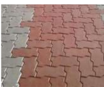
Fig 8.17: Paving A variety of Concrete brick paving to allow for sensory experience and wayfinding
