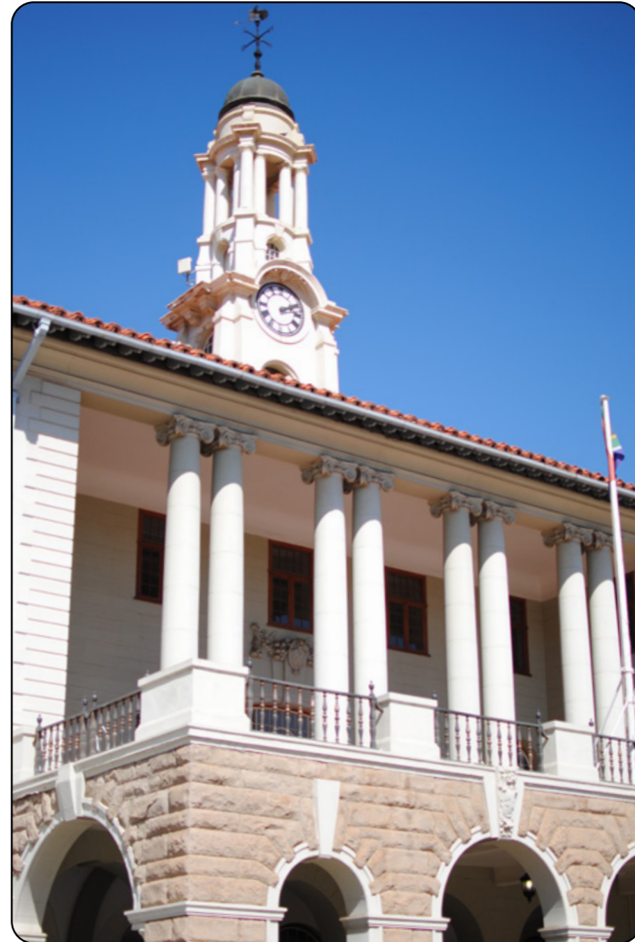
Fig. 4.57: Entrance facade of the Old Station (Ullrich 2020)
