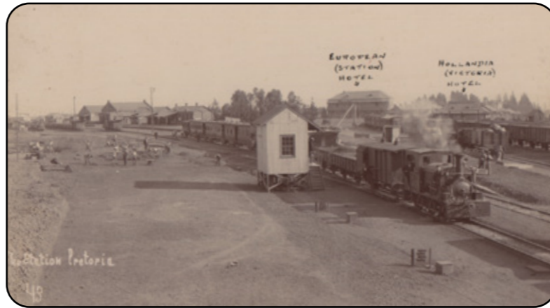
Fig. 4.62: Arrival of train at Old Pretoria Station (UPSpace c1899)
