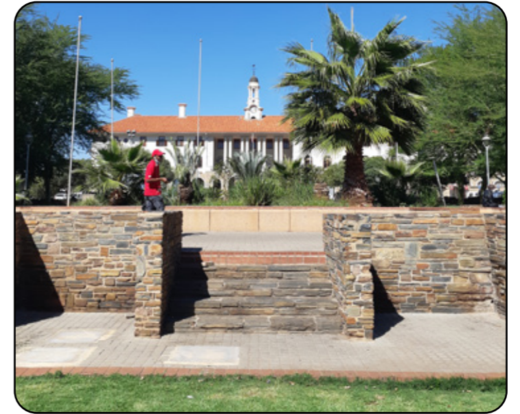
Fig. 4.58: Forecourt slate-stone retaining wall (Ullrich 2020)
