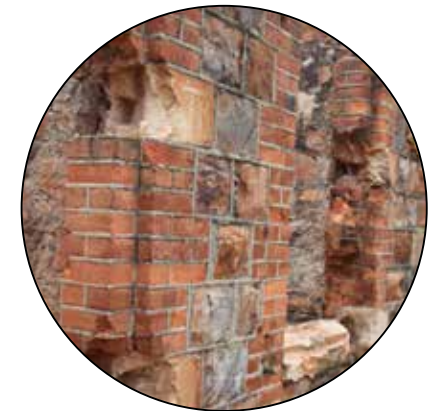
Steel, Clay Brick + Stone
