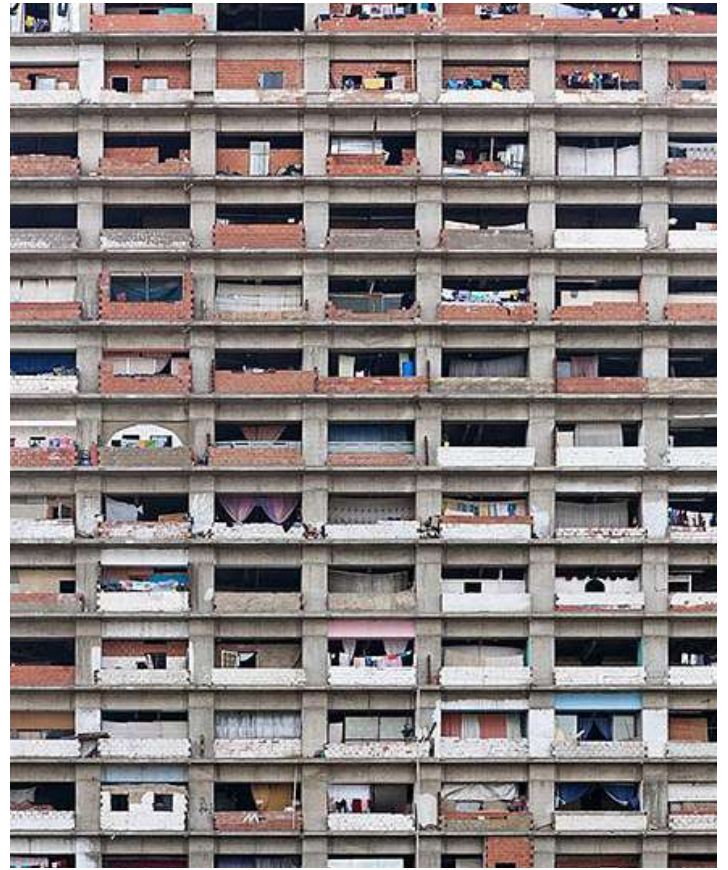
Figure 2.32 Facade infill (U-TT 2012).
