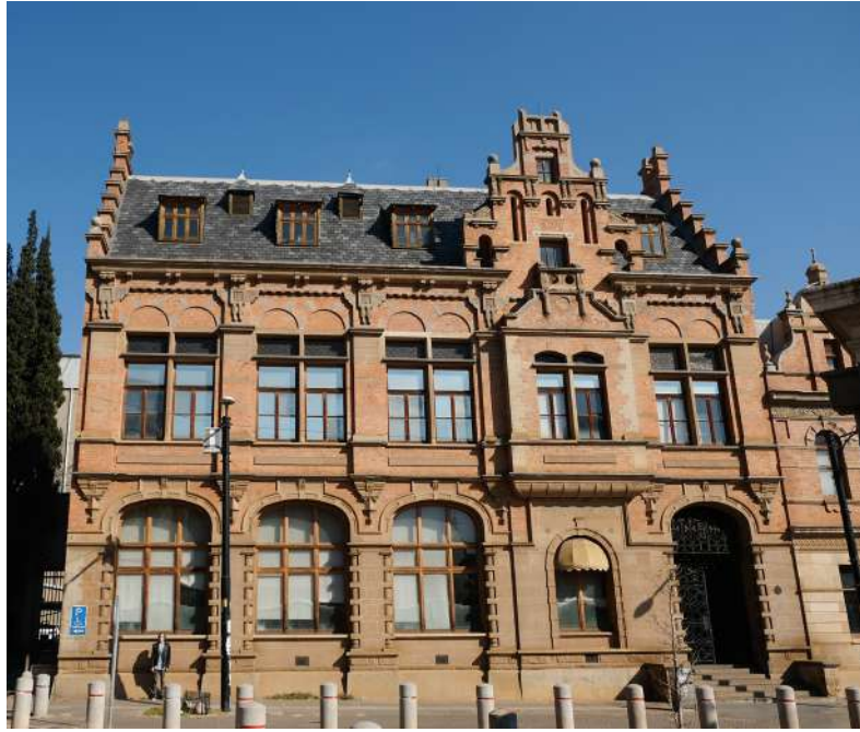
Figure 5.6 Old Netherlands Bank Front Facade (Author 2020).
