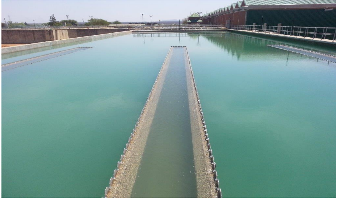
Figure 22: Plant 4 sedimentation tank overflow weirs – v-notch type
