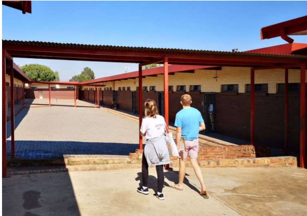
Fig. 163: Existing school hall from the outside courtyards (Greyling 2019)
