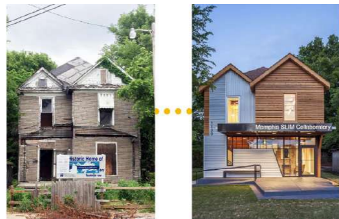
Fig. 44: Memphis Slim Collaboratory, before and after renovation by brg3s Architects (West 2014)
