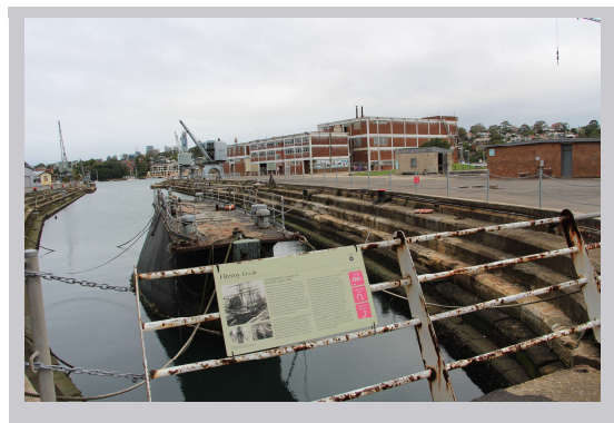
Figure 9 , Fitzroy Dock, Area R. HIP referencing the engineering technologies and techniques used in the dry dock. Emilia Zambri. 2020. Cockatoo Island
