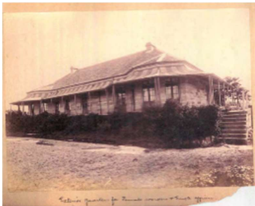
Figure 12, Biloela House. Area EFG Accommodation. Exterior Quarters for Female Warders & single officers. 1898. Dept of Corrective Services – Album H.M Gaol Biloela P22
