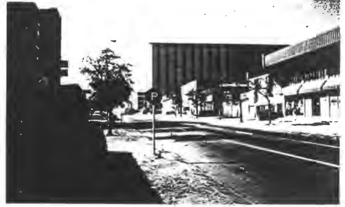
Figure 33: Pretoria West - industrial character
