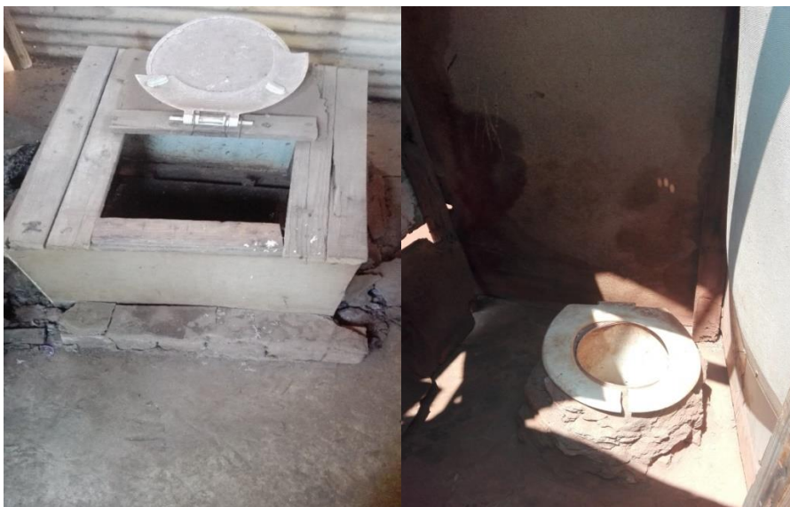
Figure 5.2: A pit latrine in Phomolong
