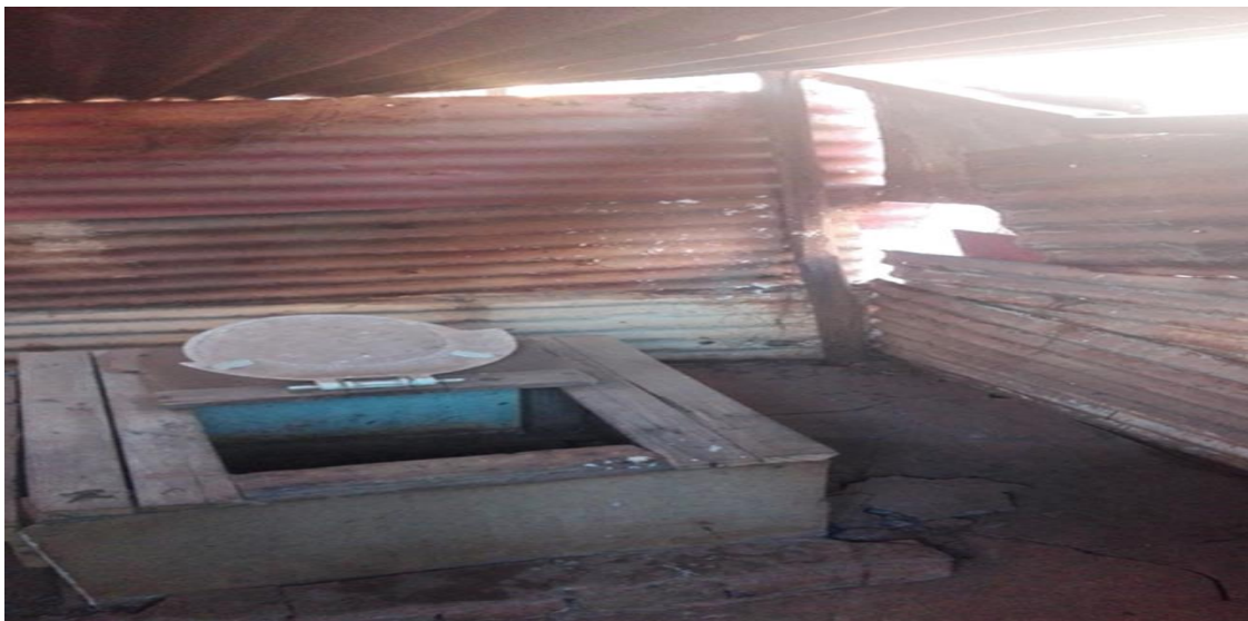
Figure 3.2: A pit latrine in Phomolong
