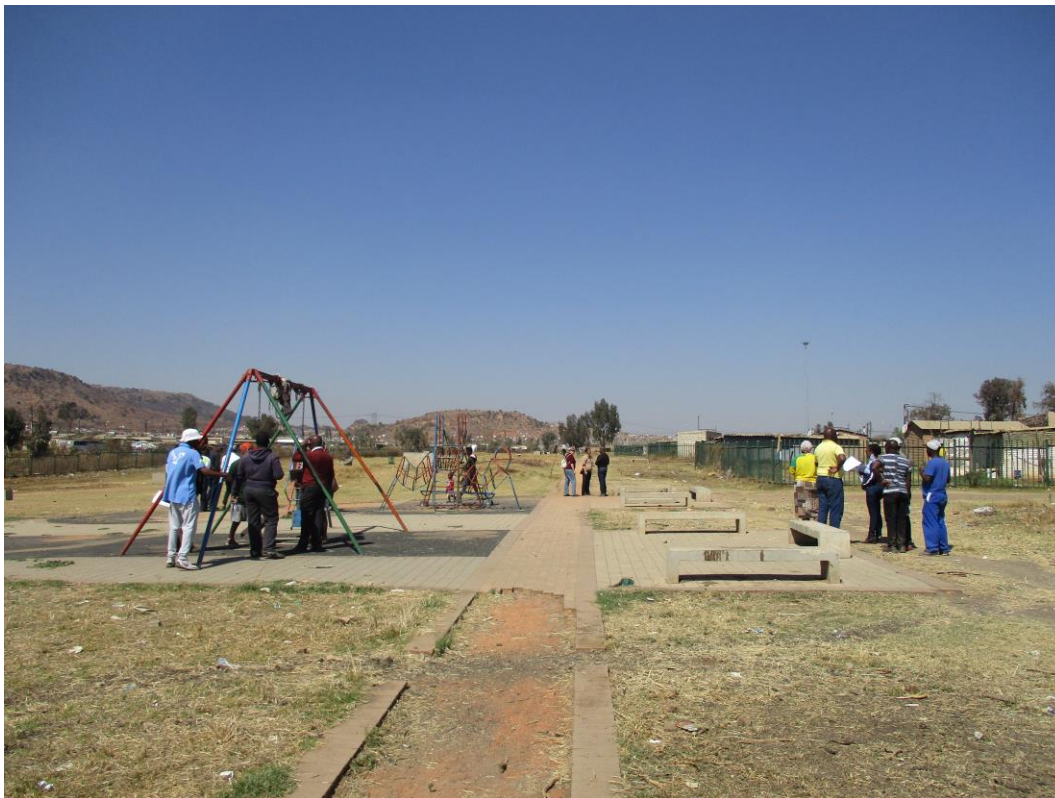
Figure 3: Broken pathway in Pienaarspoort Park
