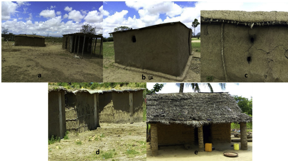
Fig. 4. Typical traditional houses in the study area, a–b shows traditional houses with iron sheet roofing, c–d shows Maasai Manyattas traditional homes and the ventilation holes in the walls thereof whilst e shows a traditional house with thatched roofing.
