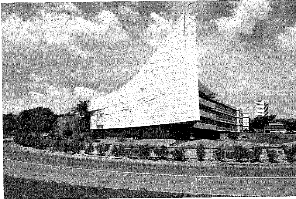
University of Pretoria building. 13 July 2014. Picture: Supplied
