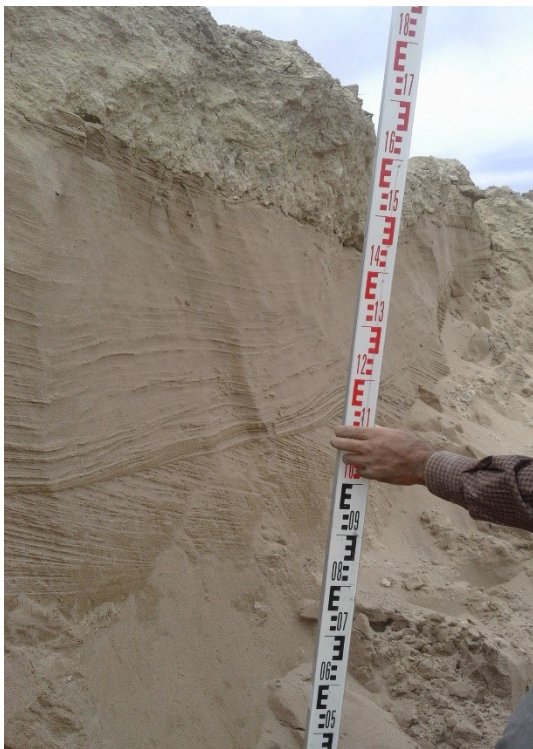
Fig 2. Excavated profile in a natural land at Zahedan Kohneh in the NC. In this profile, the Silt-clay layer that separates the surface from the subsurface is visible towards the top, with S-S sands visible beneath.
