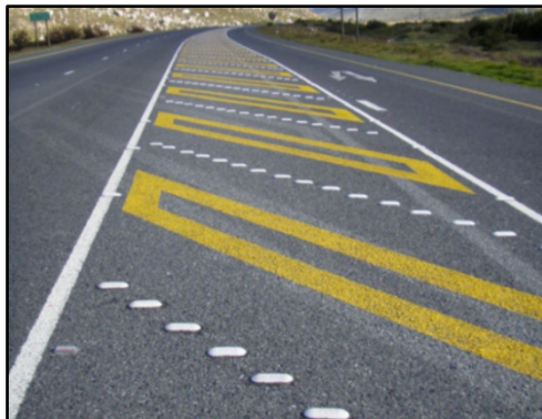
Photograph 6: Raised Speed Bump Blocks Example
