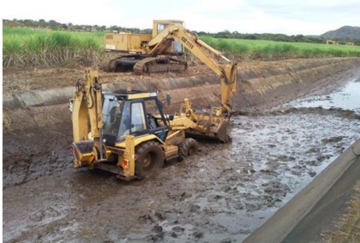
Photo 14: Large silt volumes excavated annually from the canal systems due to increasing erosion in the upstream catchment.
