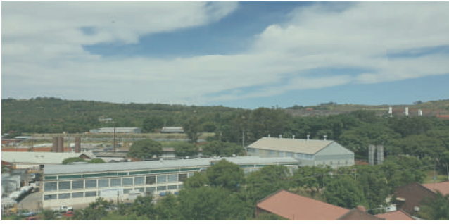
Figure-25: Looking south towards the Vibro Aggregate Mine, over the SAPS Tshwane Police Academy.
