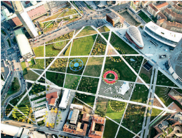
Figure-60: Aerial view of implemented project.
