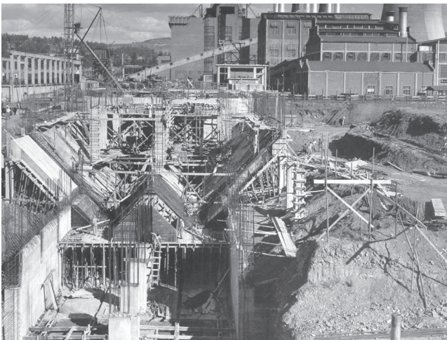
Figure-17: Showing a construction of coal bunker on northern section of the site with station A and B in the distant background. (Courtesy of the Pretoria West Power Station Archives)
