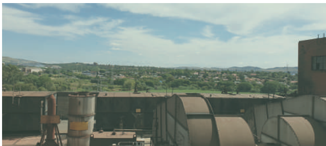
Figure-28: The View Looking west towards the suburb of Proclamation Hill.
