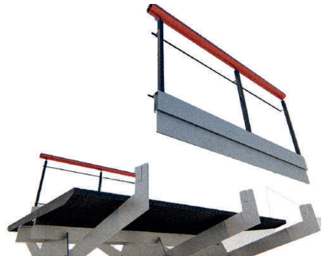
Figure-169: Step 8- Placement of pre-assembled balustrade support structures.
