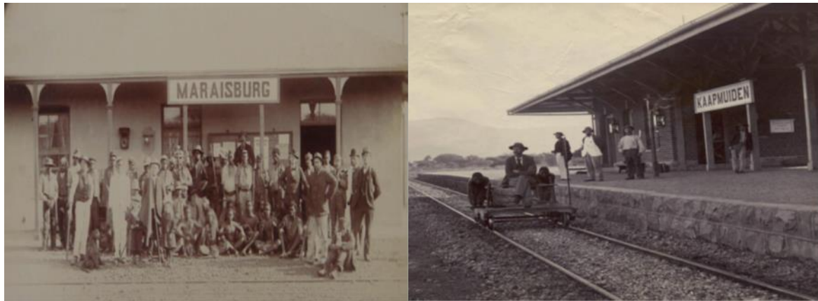
Picture 2: Image taken 1895 of NZASM personnel at Maraisburg Station; Picture 3: Kaapmuiden Station on the Eastern Line 1893 - from Pretoria to Delagoa Bay. 189
