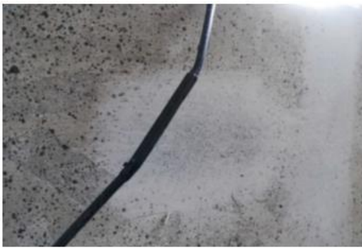
a) Preparation of concrete surface
