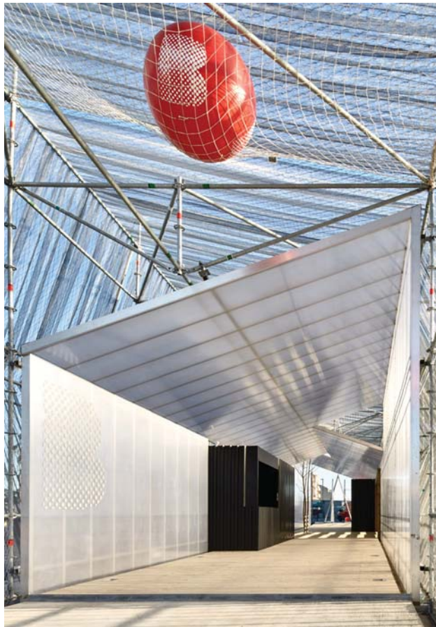
Figure 6.4.1.3 - The pavilion polycarbonate interior skin (Archdaily, 2016)
