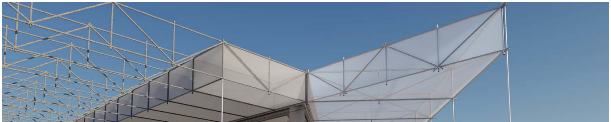
Figure 7.5.1.2 - Scaffold and polycarbonate on market pavilion (Author, 2019)
