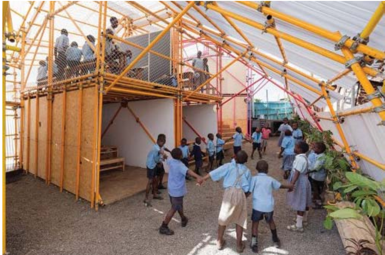
Figure 6.4.1.6 - The interior of the scaffold and polycarbonate pavilion (Iwan Baan, 2016)
