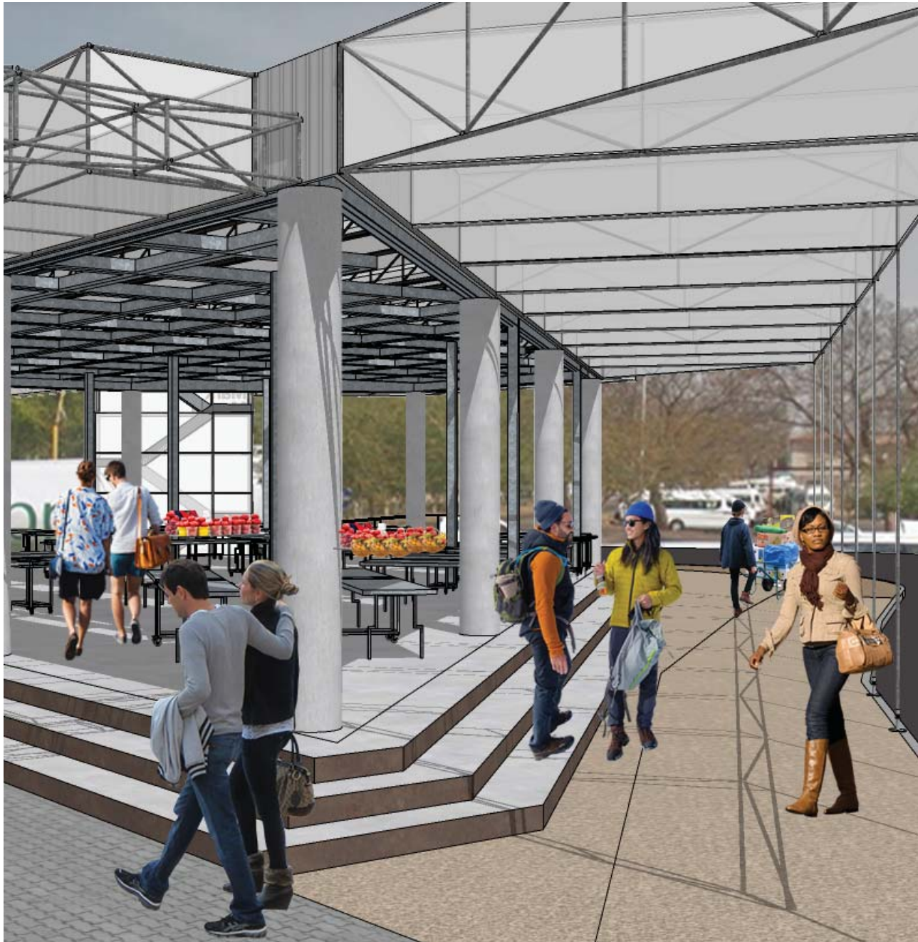
Figure 6.6.2.7 - Digital visualization of market canopy constructed of tubular steel scaffold and polycarbonate infill (Author, 2019)
