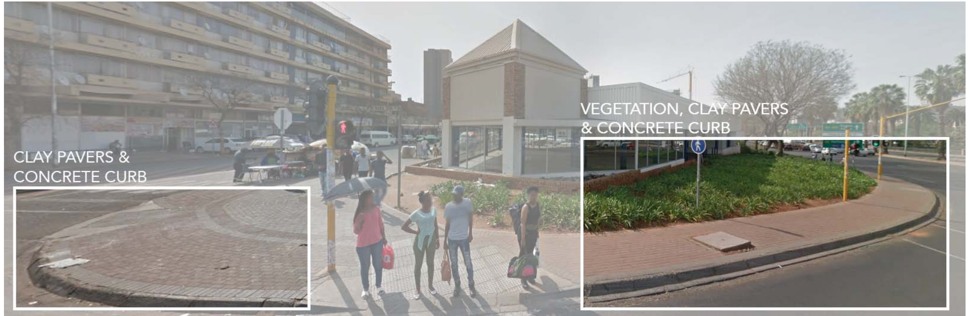
Figure 2.4.25 - Edge conditions observed from northeastern site corner. Edge consists of concrete paver sidewalks with concrete curbs (Google Earth)
