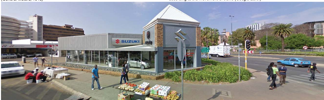
Figure 2.4.21 - The dealership is shaped to face traffic and according to the orientation of displaying vehicles (Google Earth)
