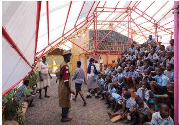
Figure 6.4.1.8 - Scaffold and polycarbonate interior (Iwan Baan, 2016)
