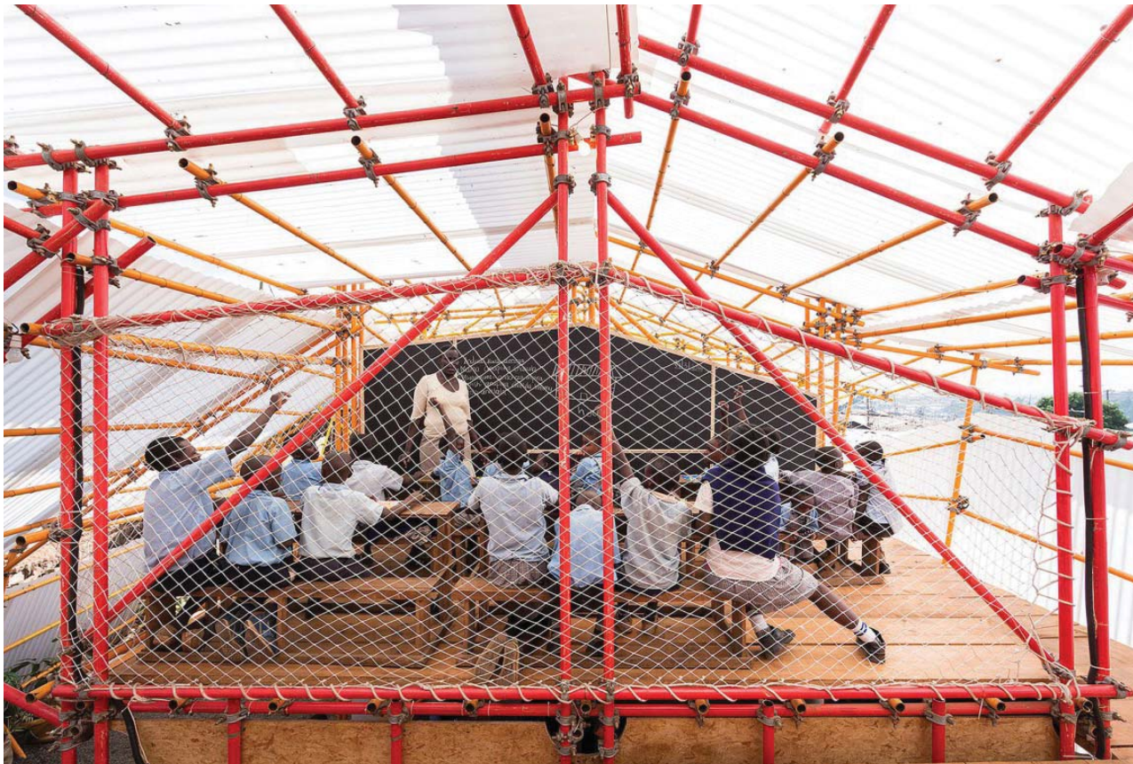
Figure 6.4.1.9 - Interior of the first floor (Iwan Baan, 2016)
