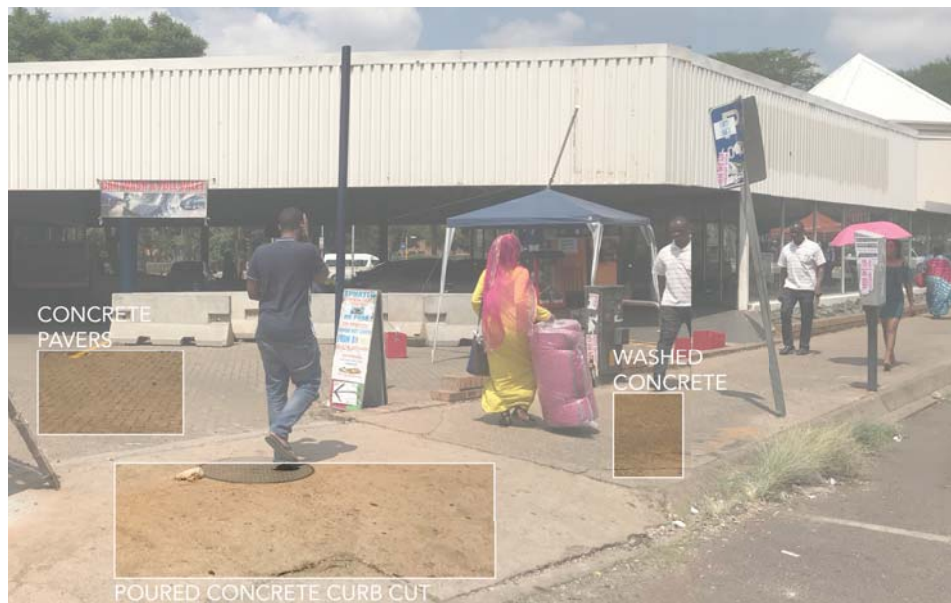
Figure 2.4.26 - Edge conditions observed on western facade. Edge consists of washed concrete sidewalk and a poured concrete curb cut for vehicular access (Author, 2019)
