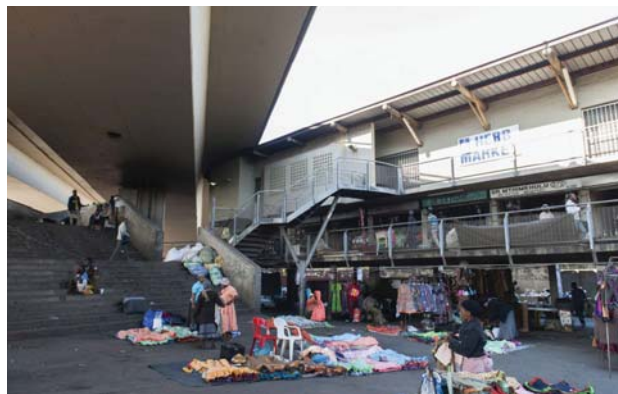
Figure 5.6.5 Warwick Junction herb market (The KwaZulu-Natal Institute for Architecture, n.d)
