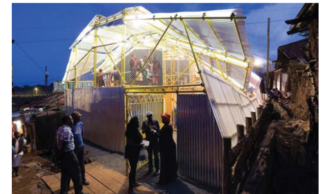
Figure 6.4.1.10 - In the evenings, the lighting design of the new school creates a landmark (Iwan Baan, 2016)
