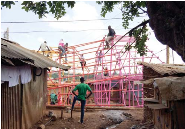
Figure 6.4.1.7 - Construction of the new school structure by locals (Iwan Baan, 2016)
