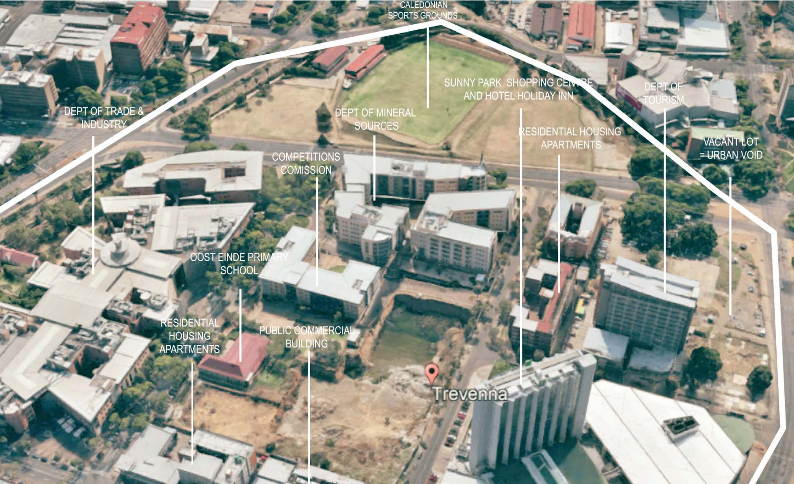
Fig 3.24: Aerial Photograph Trevenna.
