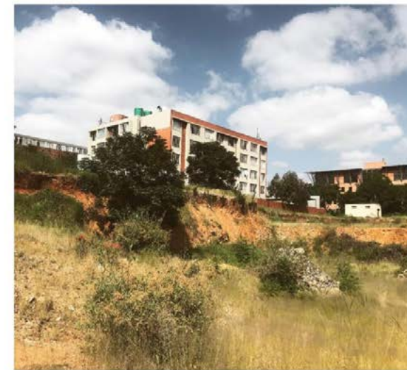
Fig 8: 75 Meintjies, dilapidated Site (Author 2019)
