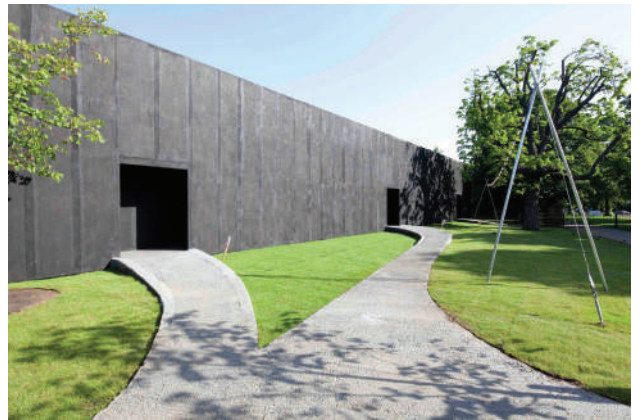
5.18 The entrance to the Serpentine Gallery Pavilion (Frearson, 2011).
