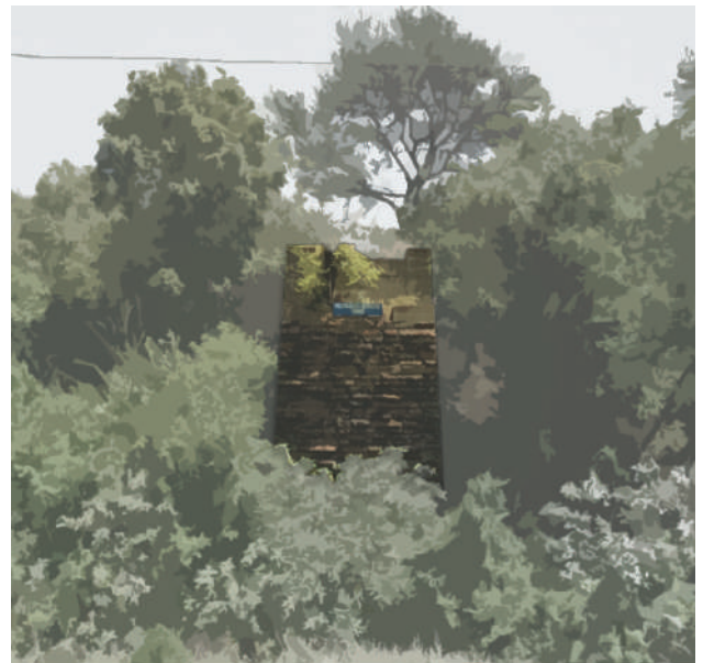
3.22 The NZASM bridge ruin (Author, 2019).
