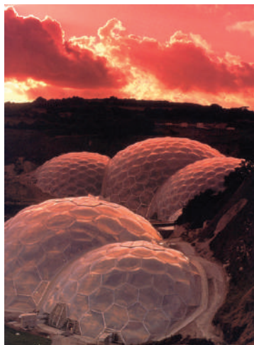
2.8 The Domes are constructed with transparent 'windows' in each hexagon and pentagon are made of ethylene tetrafluoroethylene copolymer plastic lining which is inflated (Grimshaw, 2001).
