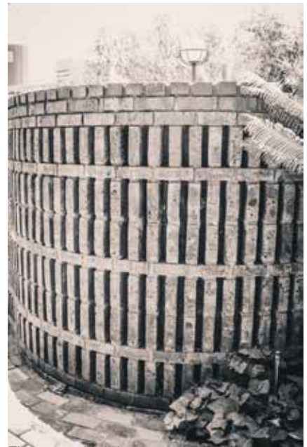
Figure142: Lighting at entrance (Author 2019)
