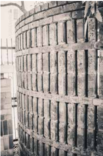
Figure140: Roof connection, Little Theatre (Author 2019)
