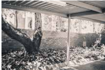
Figure126: Church boundary wall (Author 2019)
