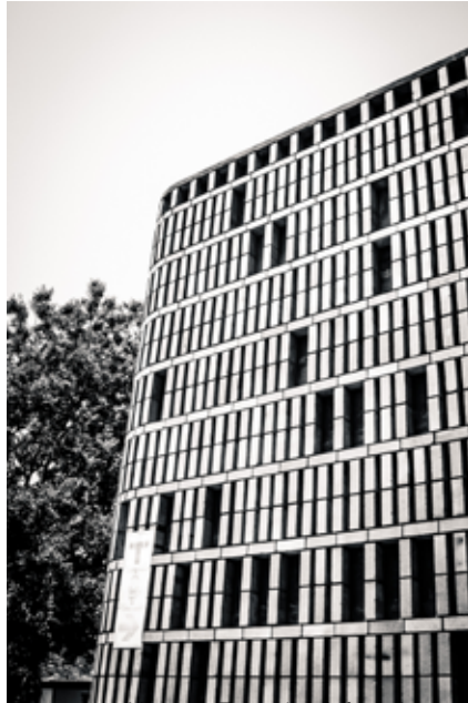
Figure147: Norman Eaton brick facade (Author 2019)
