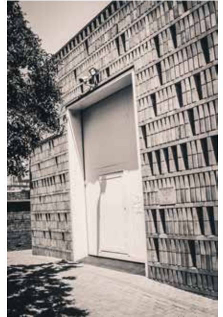
Figure148: Stage services entrance (Author 2019)
