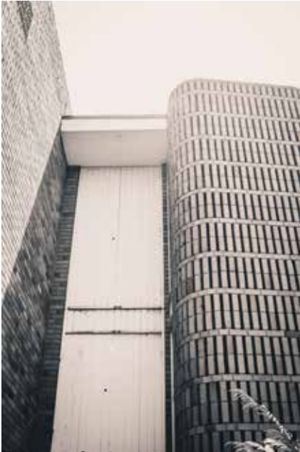
Figure146: Services entrance wall (Author 2019)
