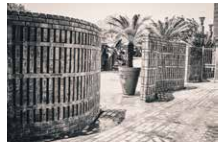
Figure136: Gap in undulating wall (Author 2019)
