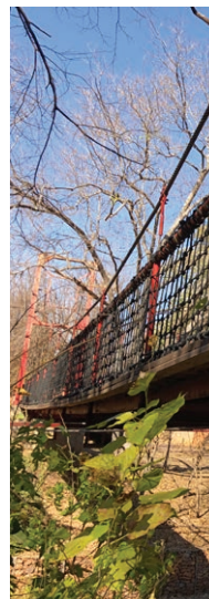
Figure 56: Suspension bridge connecting western side of site (Author, 2019)
