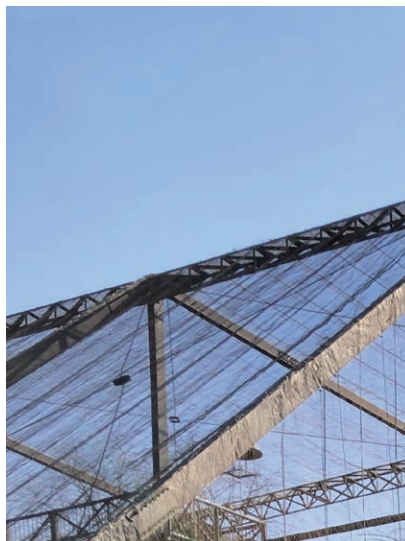
Figure 55: Aviary steel structure
