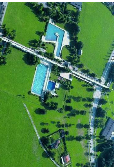
Figure 5.7: Bellinzona Bathhouse aerial photograph – Aurelio Galfetti, Flora Ruchat-Roncari (www.Hiddenarchitecture.net, 2019)
