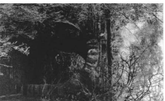
Figure 2.35: Photograph by R. C. de Jong of Old arched culvert under the previous NZASM railway (Pretoriana no. 091, 1987)
