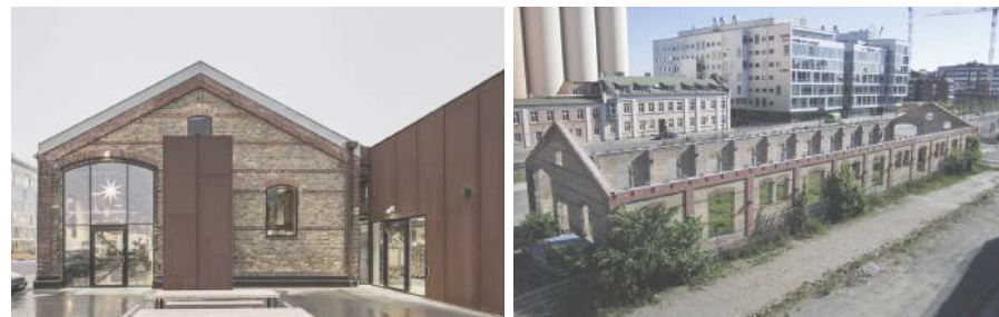
Figure 2.17 & 2.18 Exterior of Market hall, (Pihl 2019)
