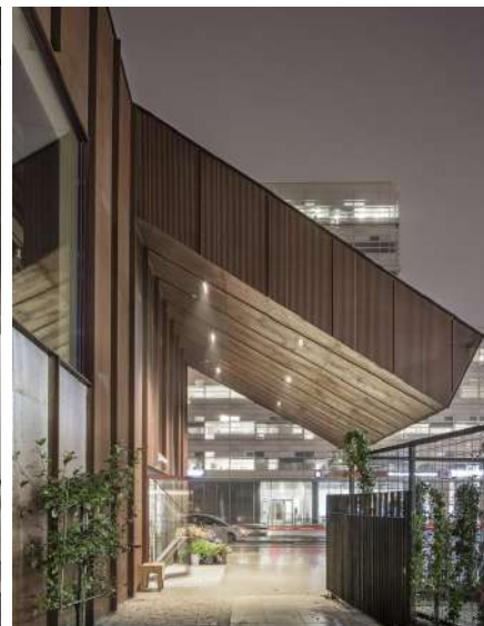
Figure 2.20 Roof overhang of the new extension, (Pihl 2019)
