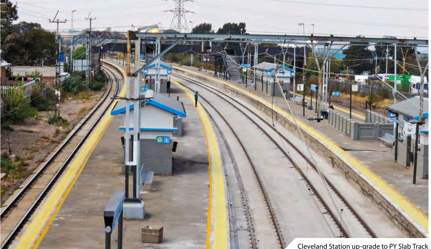
Cleveland Station up-grade to PY Slab Track
