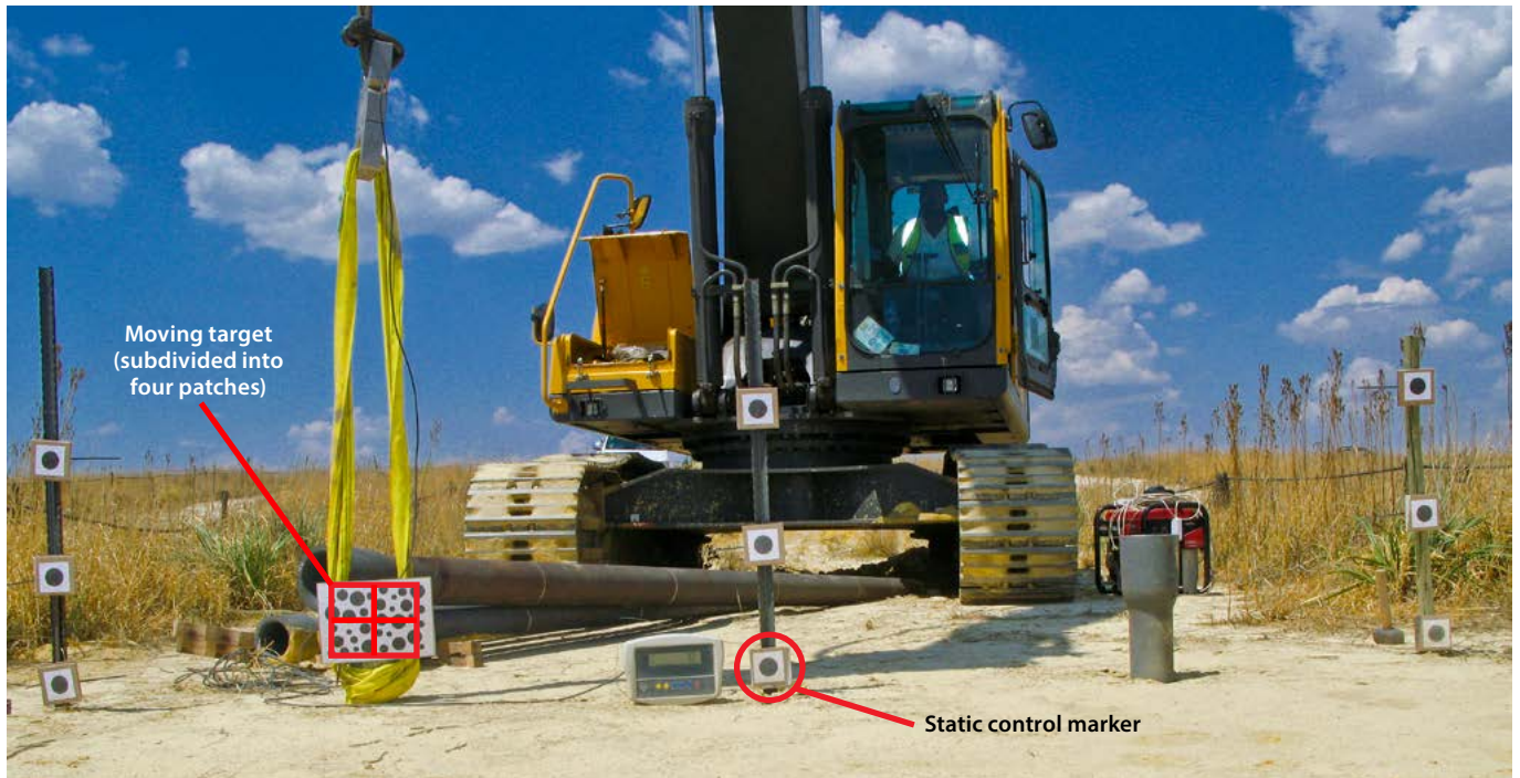
Figure 2 Typical image used for tracking pile displacement
