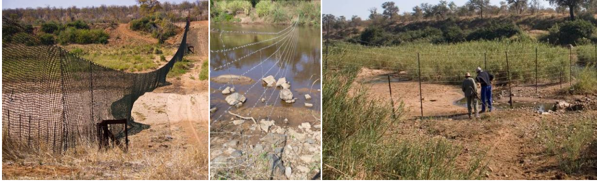
Figure 5.2. Three examples of fence river crossings: A net across a large river (Letaba) and two sacrificial fences with varying degrees of reinforcement
