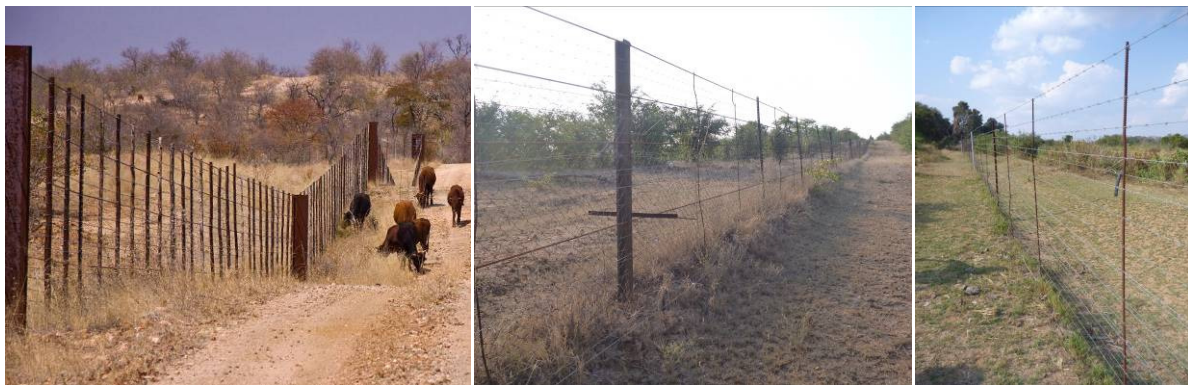
Figure 5.1. The three fence types considered (from left to right): I-beam and cable; Railway line and cable and Game fence.
