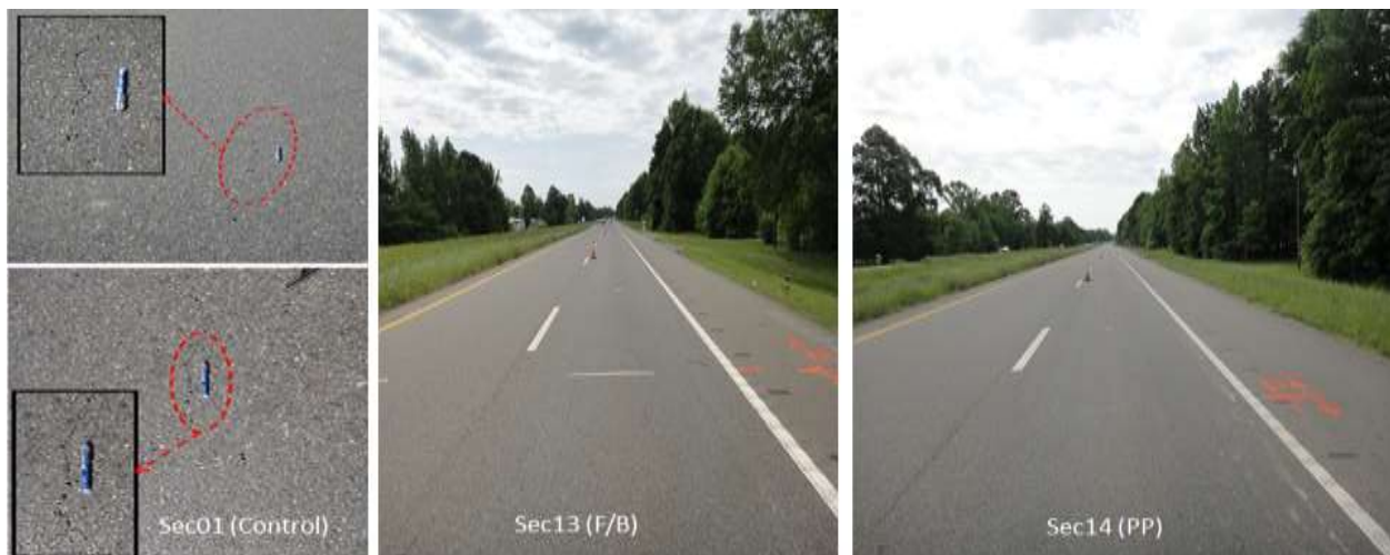
Fig. 11. Pictorial Surface View of the US 59 Test Sections.
