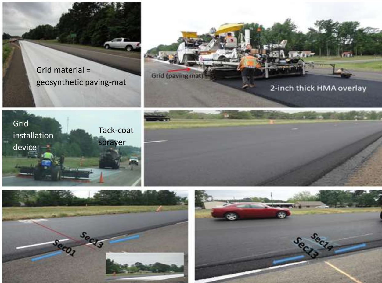
Fig. 4. Geosynthetic Installation and HMA Overlay Construction.
