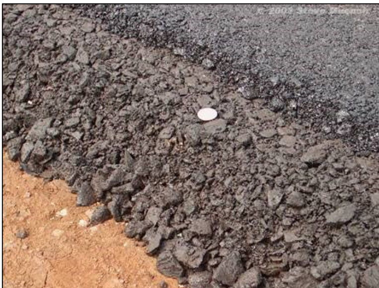
Figure 2-19: Typical bitumen treated base (Pavement Interactive, 2012a).
