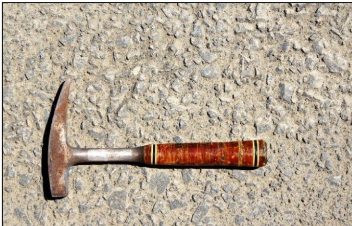
Figure 2-14: Completed, slushed G1 base (Kleyn, 2012).
