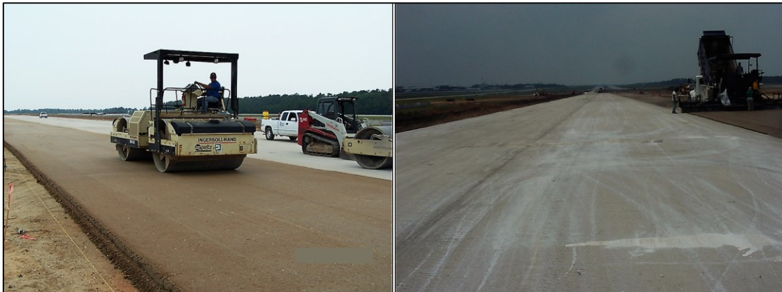
Figure 2-18: Typical cement treated base (AG Peltz, n.d.).
