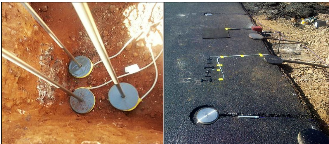
Figure 3-3: Emu strain coils, pressure cells, big mat stress sensors, and strain gauges.
