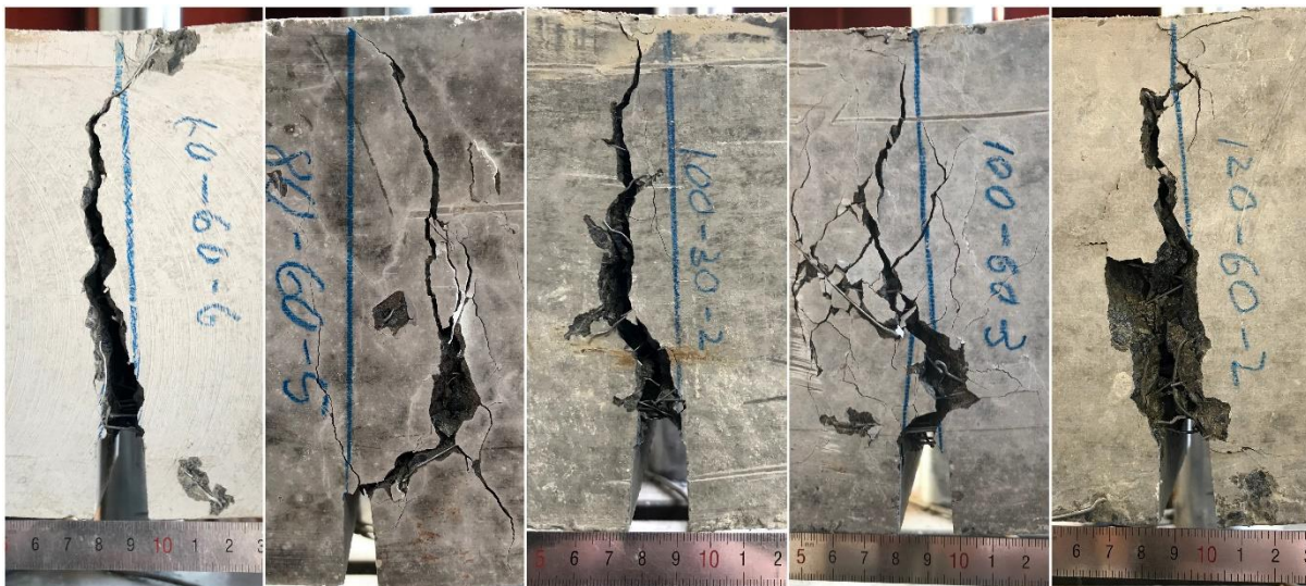
Figure 4-11: Examples of various observed crack patterns
