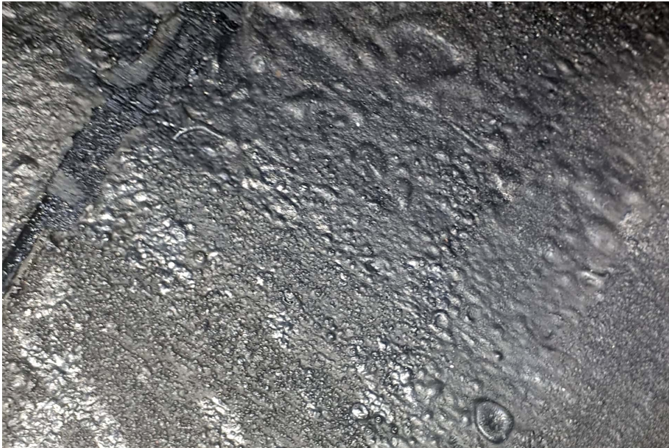
Figure A.4: The inside surface of the still after a couple months of operation, showing the deterioration of the Durapond sealant.
