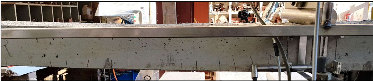
Figure B. 14: Crack spacing along right span during testing
