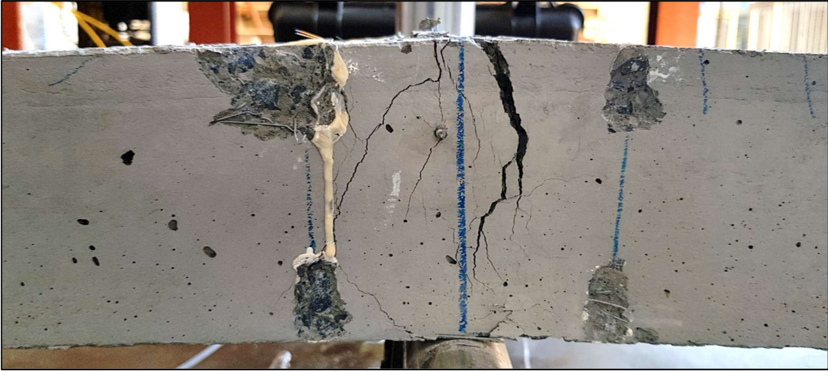
Figure B. 32: Crack formation above centre support after testing
