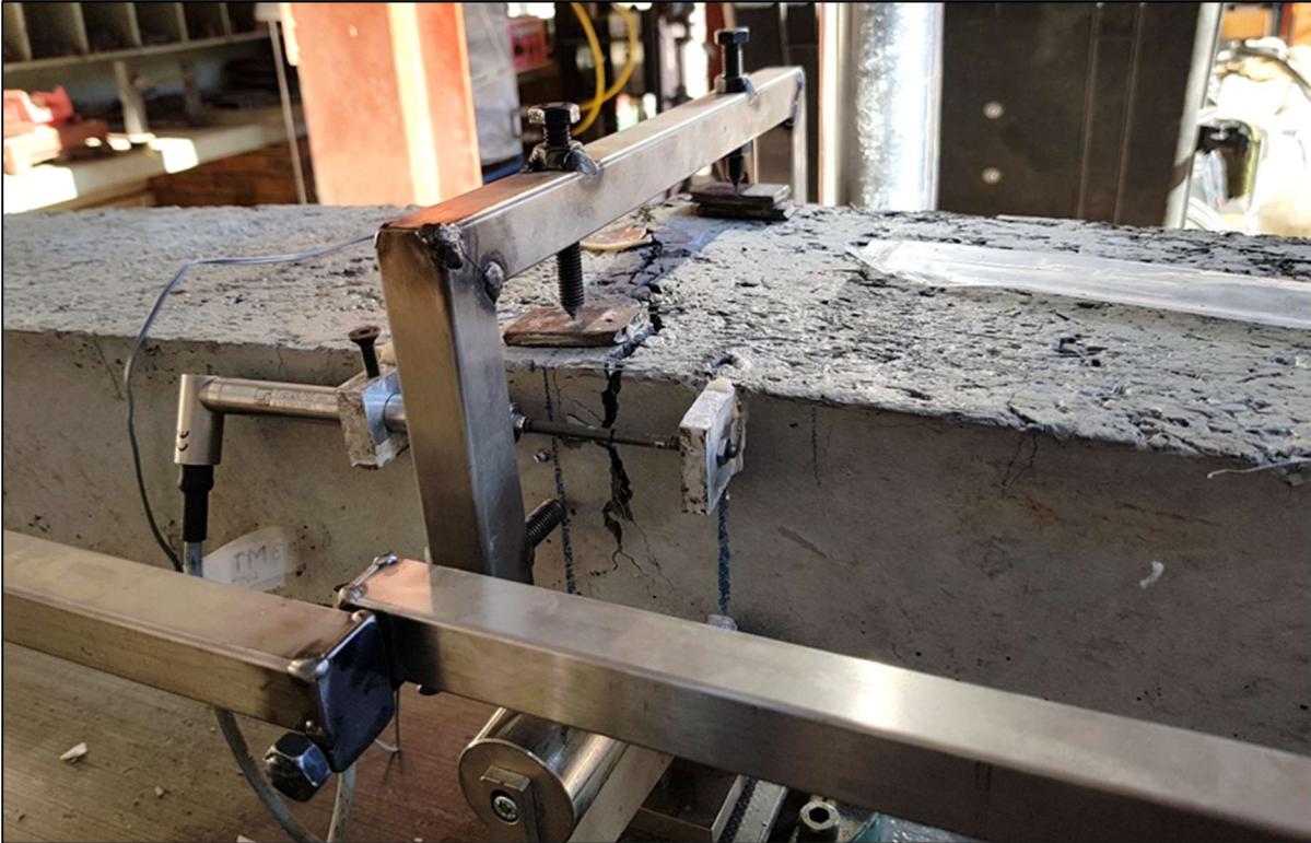
Figure B. 24: Crack formation above centre support during testing
