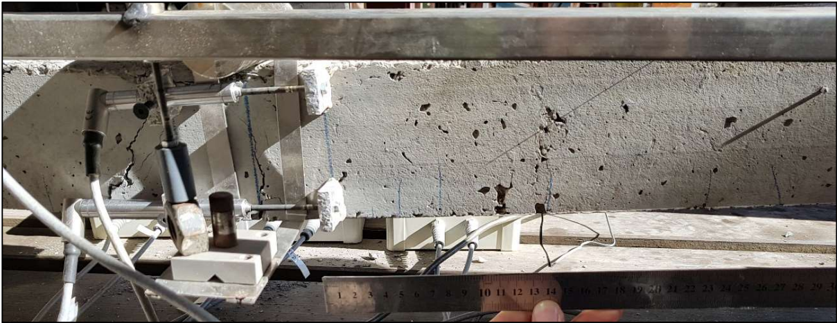
Figure B. 26: Crack spacing along left span during testing
