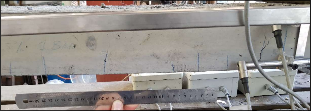
Figure B. 19: Crack spacing along right span during testing
