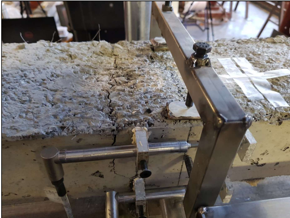
Figure B. 5: Cracking at centre support during testing
