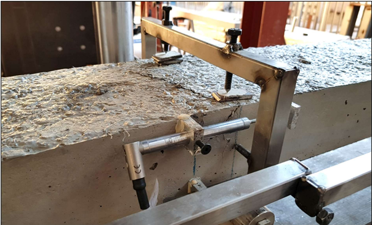
Figure B. 27: Crack formation above centre support during testing
