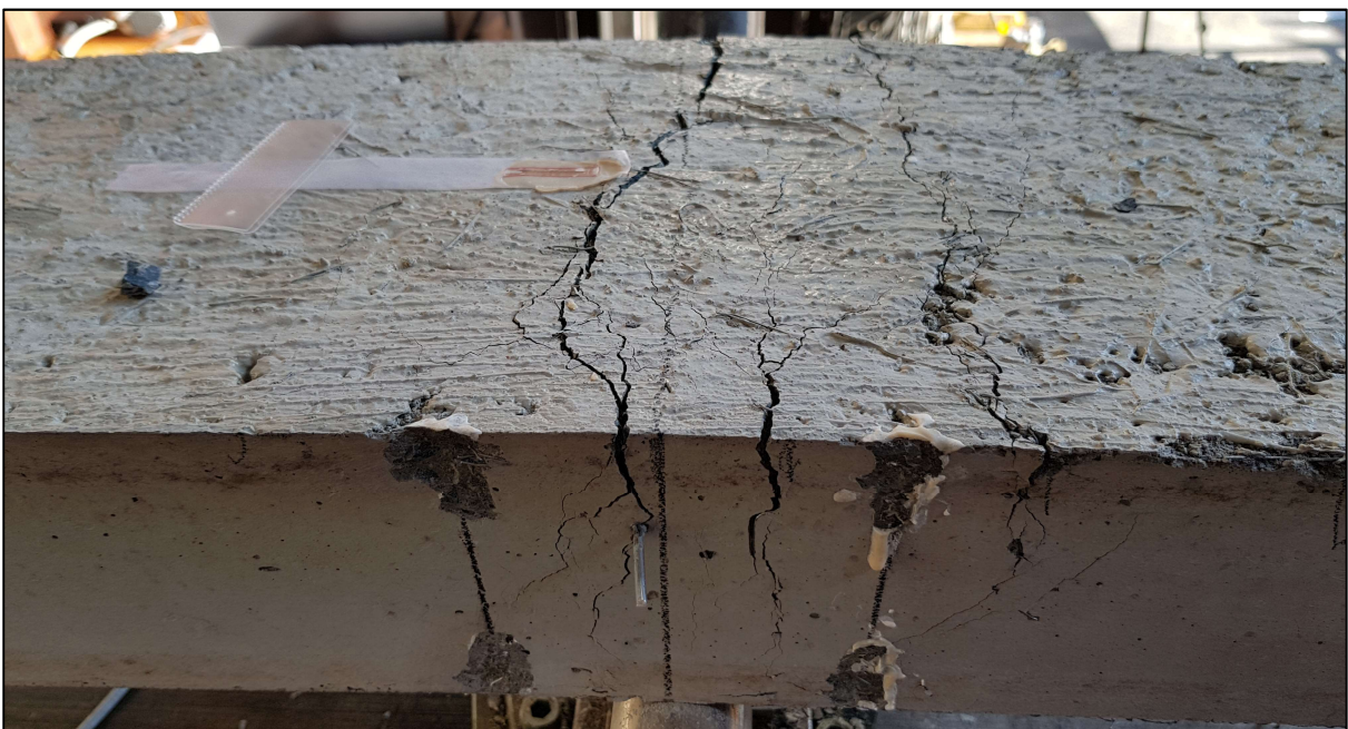
Figure B. 12: Cracked section at the centre support after testing
