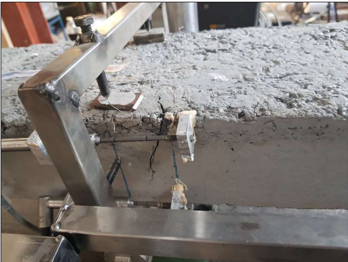
Figure B. 17: Cracking above centre support during testing
