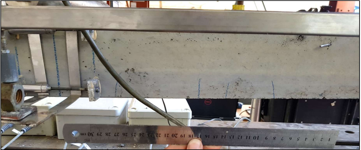
Figure B. 20: Crack spacing along left span during testing
