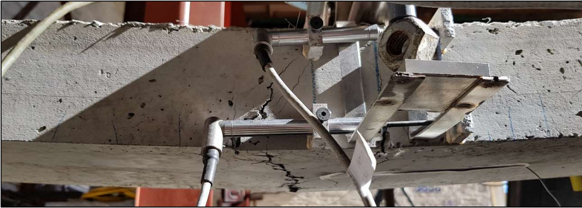
Figure B. 25: Crack formation along right span during testing
