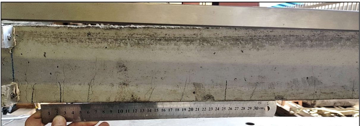
Figure B. 11: Crack spacing along left span during testing
