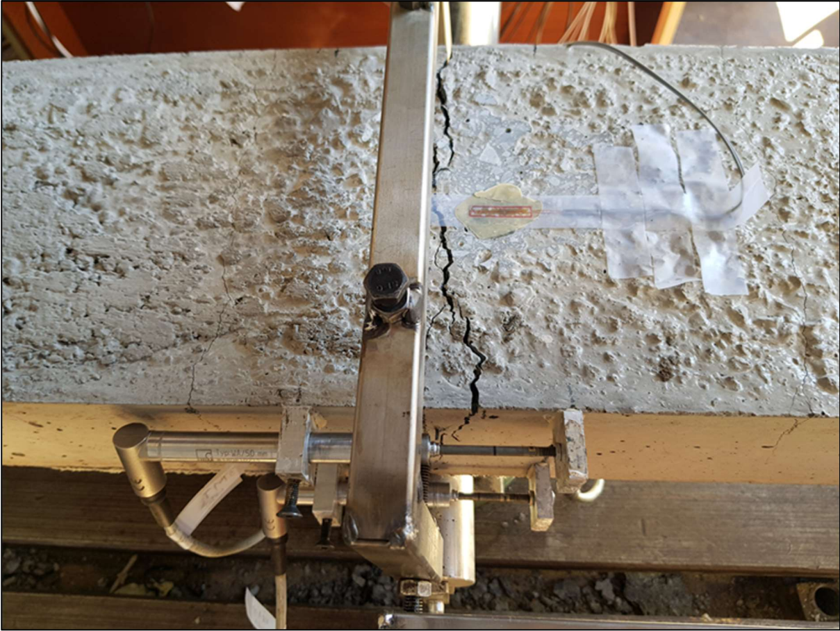
Figure B. 1: Cracked section at centre support
