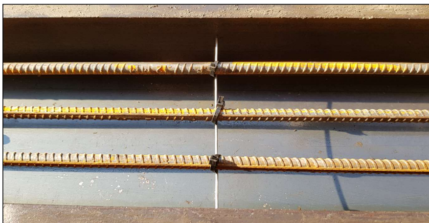
Figure 5-2: Reinforcing spacing
