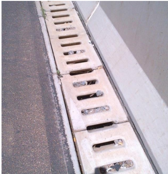
Figure 2-7: Clogging of slotted inlets (privately captured)
