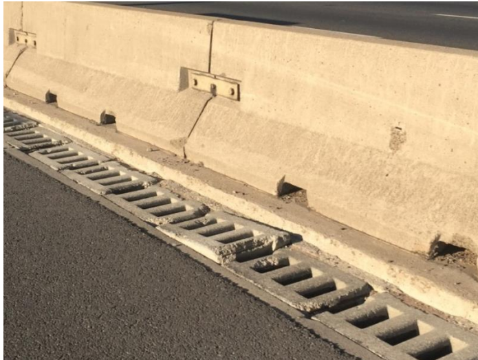
Figure 2-8: Slotted inlet cover failure and settlement (privately captured)
