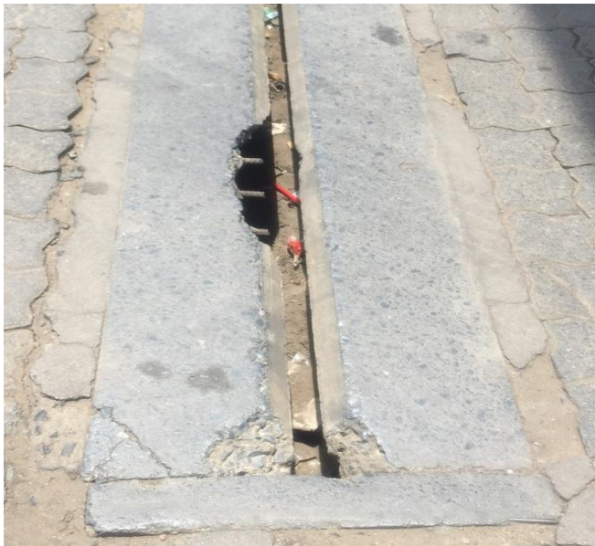
Figure 2-9: Damaged slotted inlets (privately captured)
