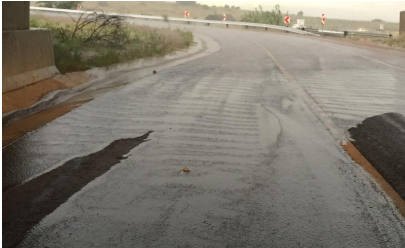
Figure 2-2: Sheet flow on the pavement surface (privately captured)
