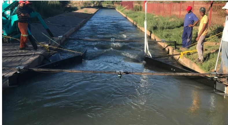
Figure 16. Narrowed canal width with installed turbine
