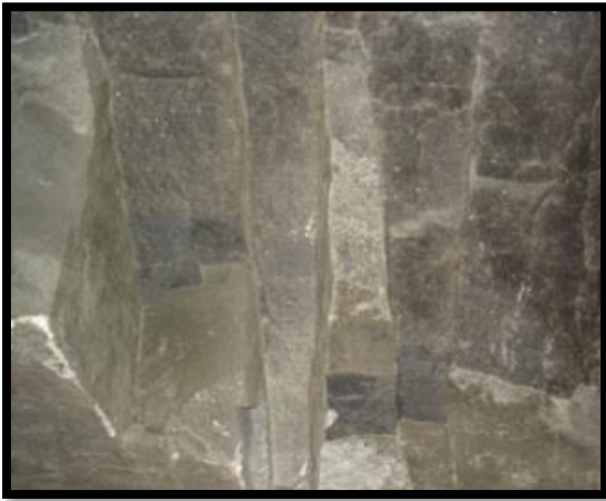
Figure 9 – Joint set within underground excavation.
