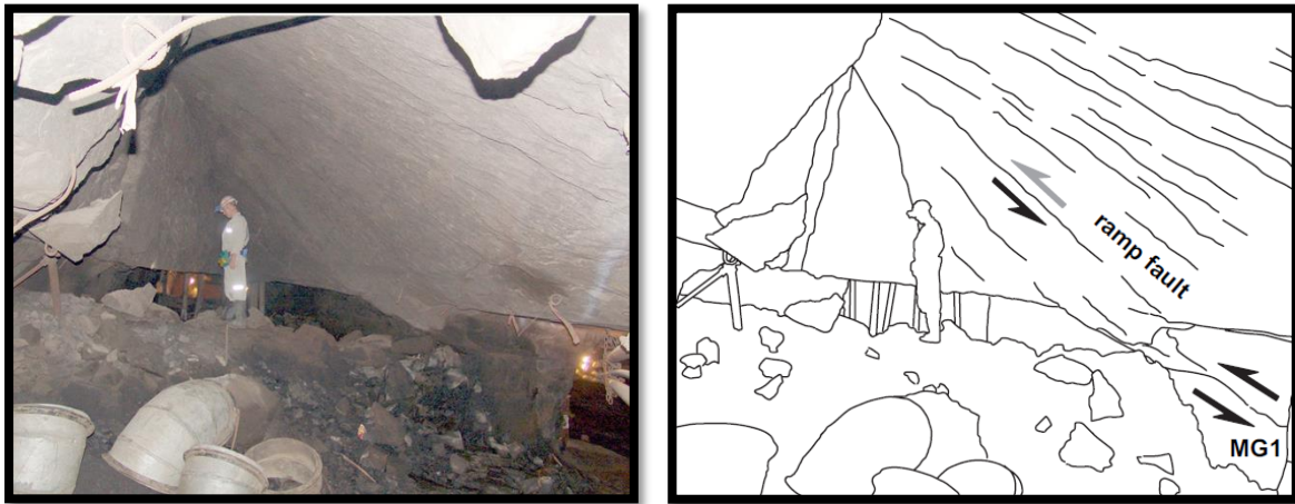
Figure 15 – Failure of “dome” thrust fault feature within underground workings (edited from (Perrit and Roberts, 2007 and Internal presentation-Glencore Alloys).
