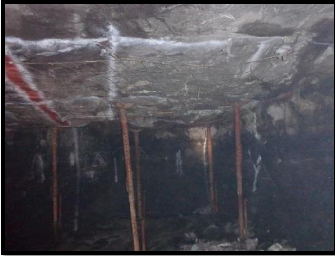
Figure 25: Temporary support with safety nets to act as support for the installation of permanent support.
