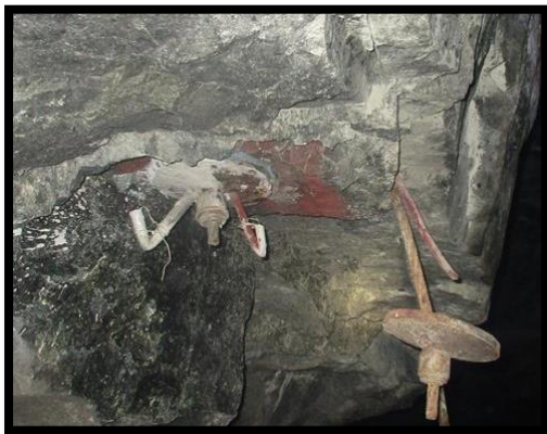
Figure 27: Grouted cable anchor support within underground workings (J, Bezuidenhout, 2017).
