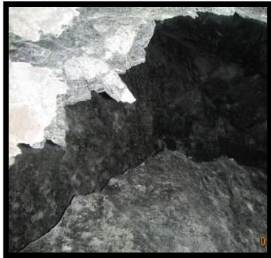
Figure 33: Photo indicating the extent of the dislodged rock and water within hanging wall rocks- Note the serpentinite coating along exposed planes.
