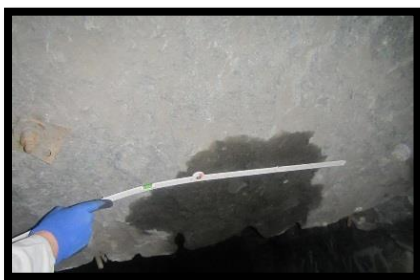
Figure 34: Photo indicating the extent of the dislodged rock and water within hanging wall rocks- Note the serpentinite coating along exposed planes.
