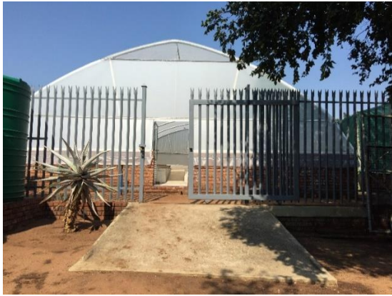
Plate 1: An external view of the trial house as viewed from the entrance.
