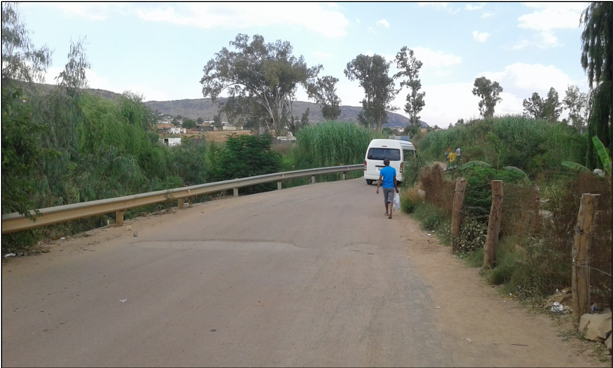
FIGURE 53: Bridge built by Stoffel Motloutsi crossing to Mahube mall on to Tsamaya Road
