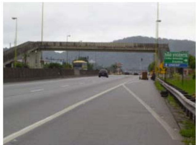
Figure 8. Second pedestrian walkway in the urbanised part of the highway.
